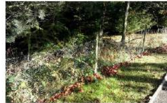
Photo Name: 14 Subject: Wire Fence Condition: Needs attention Remarks: Sagging wire.
